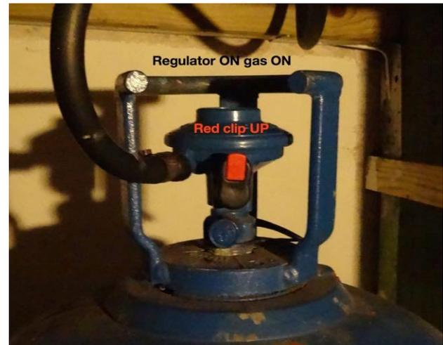
To connect the regulator; place it on the gas cylinder, lift the red clip, and turn the black knob clockwise. When the red clip points upwards, the regulator is connected and the gas is on.
